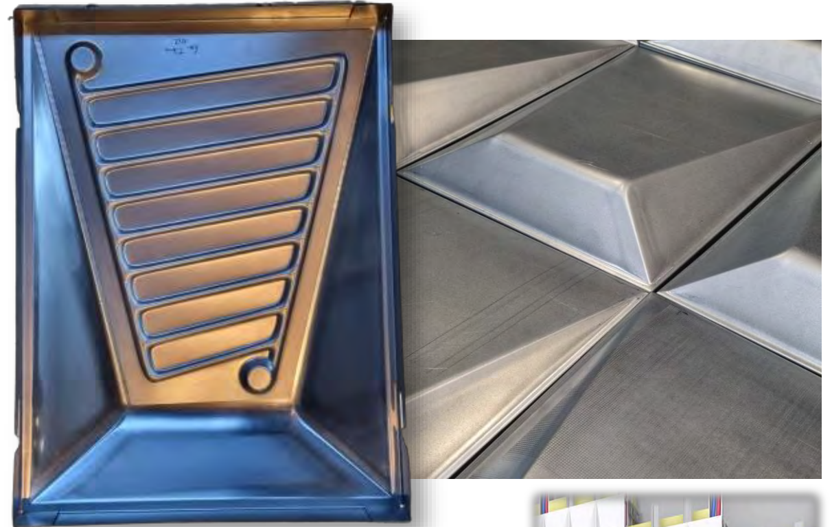
Freeform facade element with solar thermal functionality
